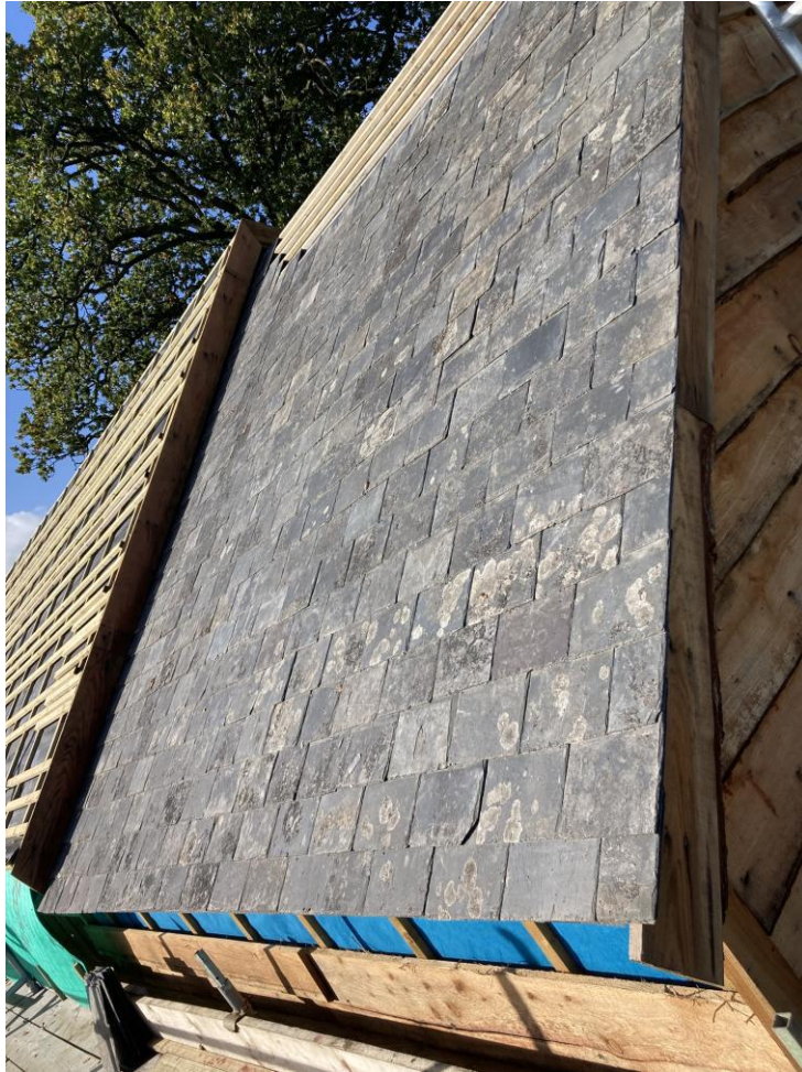
Reclaimed Welsh slates from local building of 1860 sit well on the new roof. D Maloney
