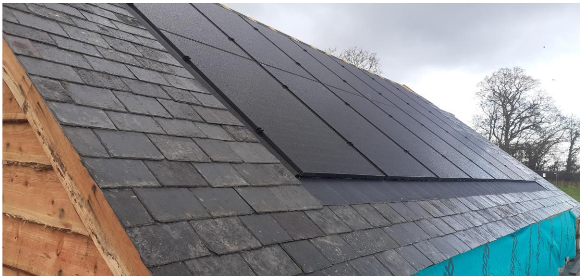
Solar panels completed and tested. H Wilson
