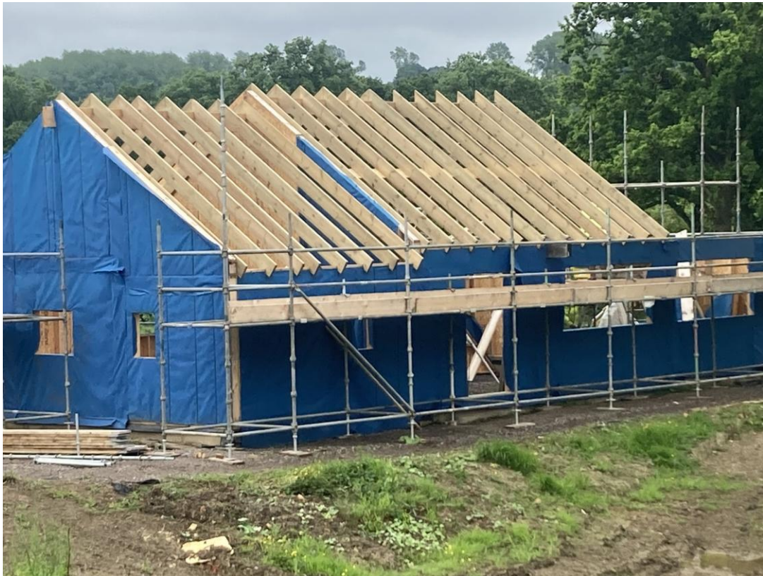
Rafters installed. D Maloney
