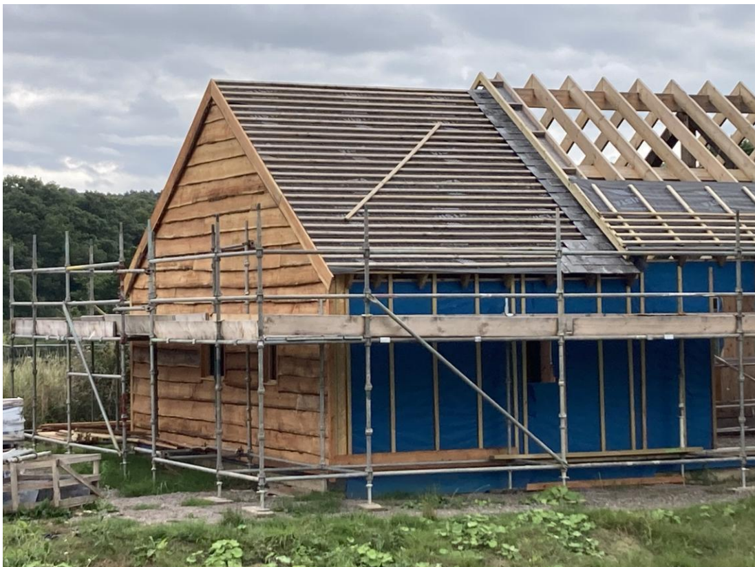
Roofing felt and batten applied. Other volunteers clad the northern end wall. D Maloney
