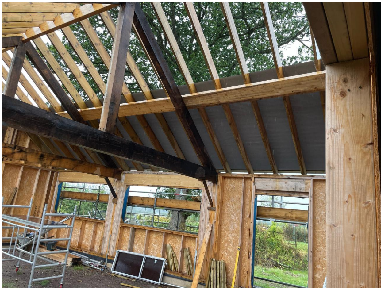
Interior walls will be insulated before being cladded which will hide the insulation. D Maloney
