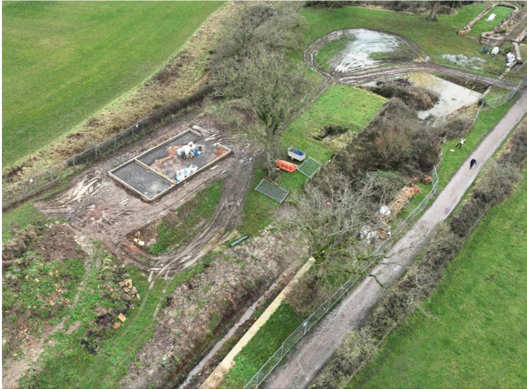
Foundations created and sole plate blocks installed. S Court
