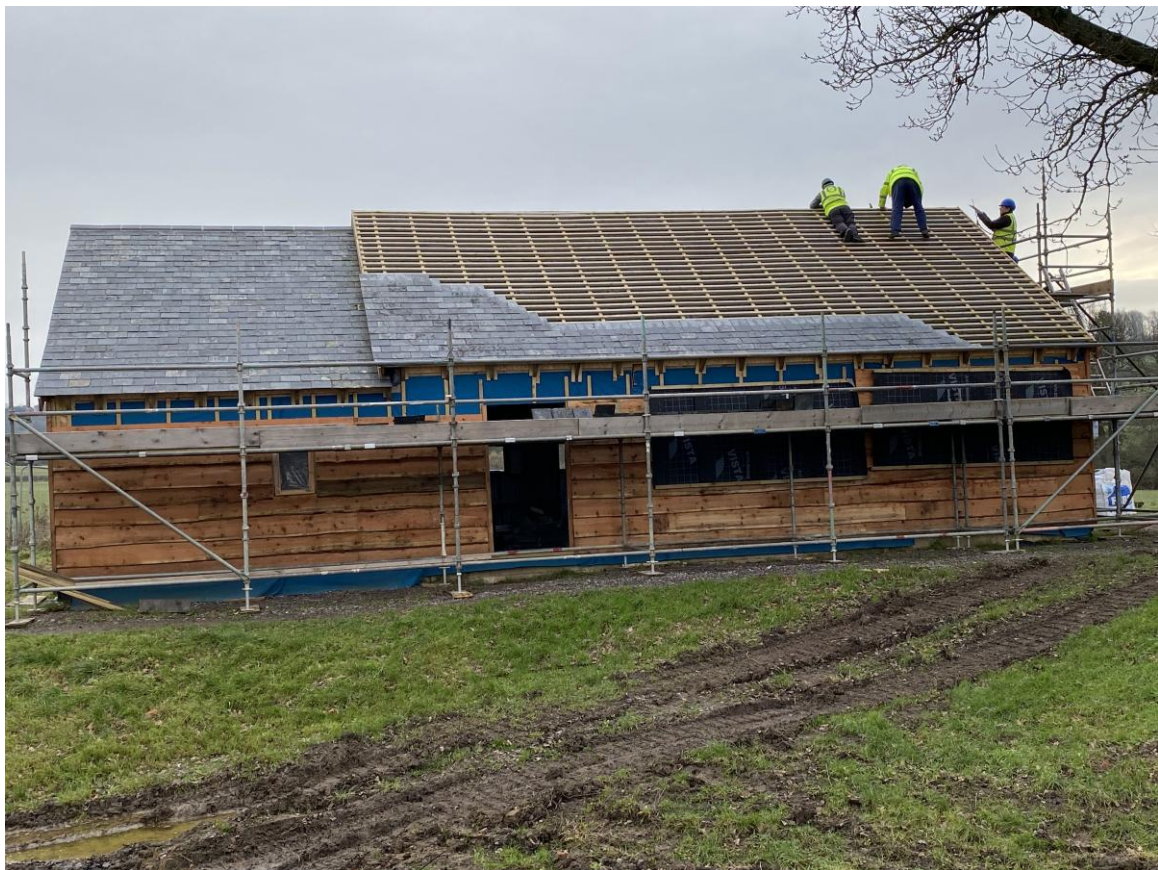
Roofing volunteers move to the west roof. Wall volunteers have cladded this side with larch from local sawmill. Larch was chosen as in 12/18 months it will start to "age" and turn shades of grey. H Wilson
