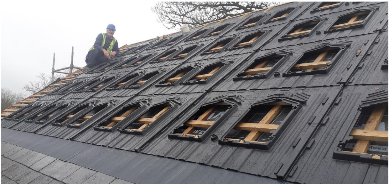
We went for a solar panel system that sits directly on the roof battens, this saving funds on Welsh slate. These trays will take the solar panels. H Wilson
