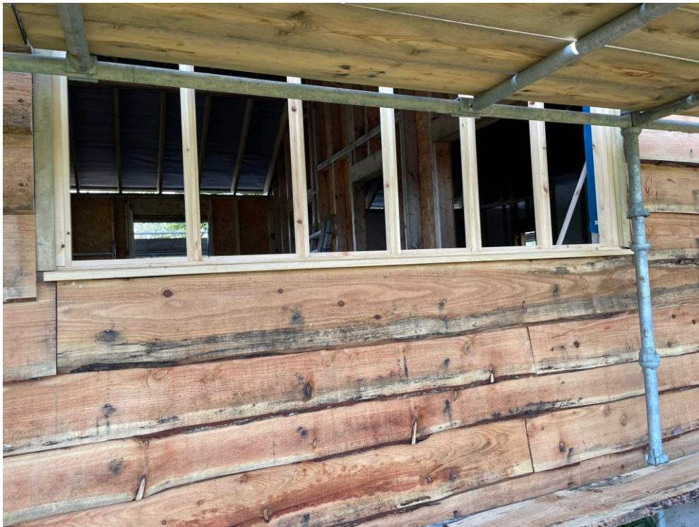
Bespoke window frames made by canal trust volunteer.
