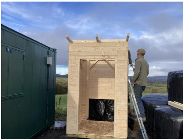
Installation of Woo GT Cabin at Solidarity Farm CIC
